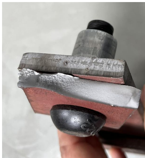
Figure 9. The fatigue failure of the connection plate
